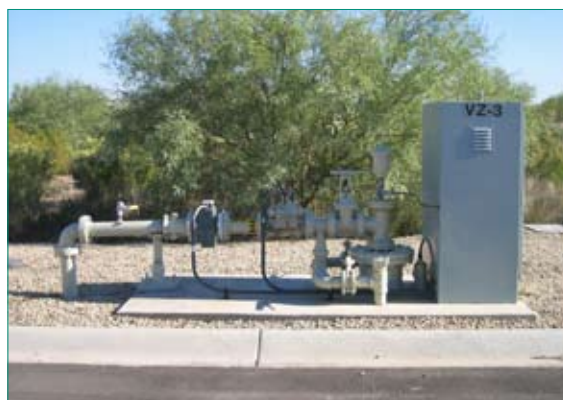
A reclaimed water recharge well in Phoenix, AZ. SOURCE: Andy Terrey, City of Phoenix.
