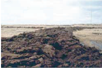
Figure 100: An area selected for natural revegetation monitoring on Shemya Island. This road is being reclaimed with a locally excavated peat overlay that is allowed to develop a vegetation cover without assistance.
