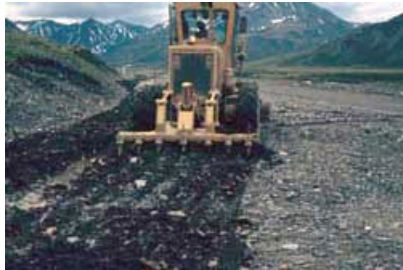
Figure 106: An area being prepared for natural revegetation by using a ripper bar on a grader. This is the final condition of the prepared surface.
