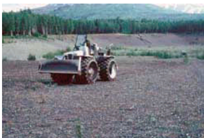
Figure 102: A landfill compacter being used to loosen and imprint the surface of an old gravel pit.
