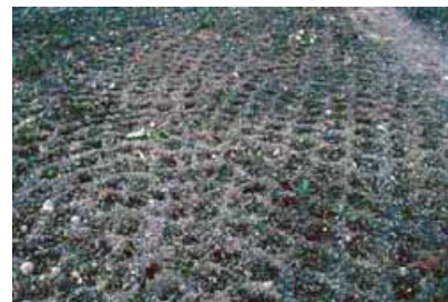
Figure 103: The imprinted pattern on the surface of the gravel pit. The pock marks trap moisture and seed. The steel wheels of the compacter (sheep’s foot) on the hard surface loosen the soil, forming a more vegetation-friendly condition.
