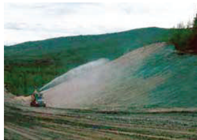
Figure 88: Hydroseeding a large-cut slope. This is the ideal area and use for a hydroseeder.
