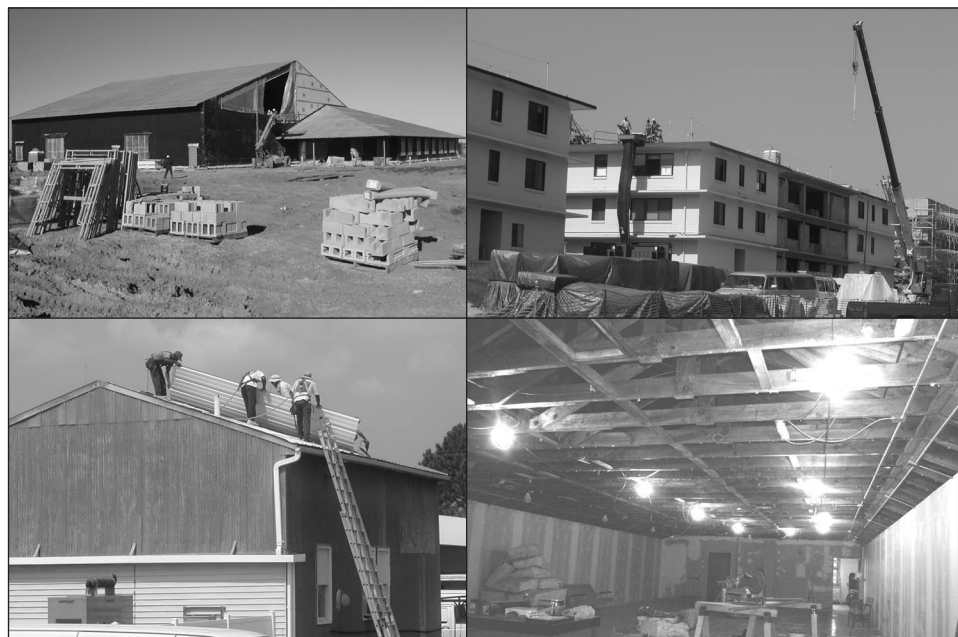
Figure 5: Typical Examples of Facility Improvements at Various Reserve Component Locations
