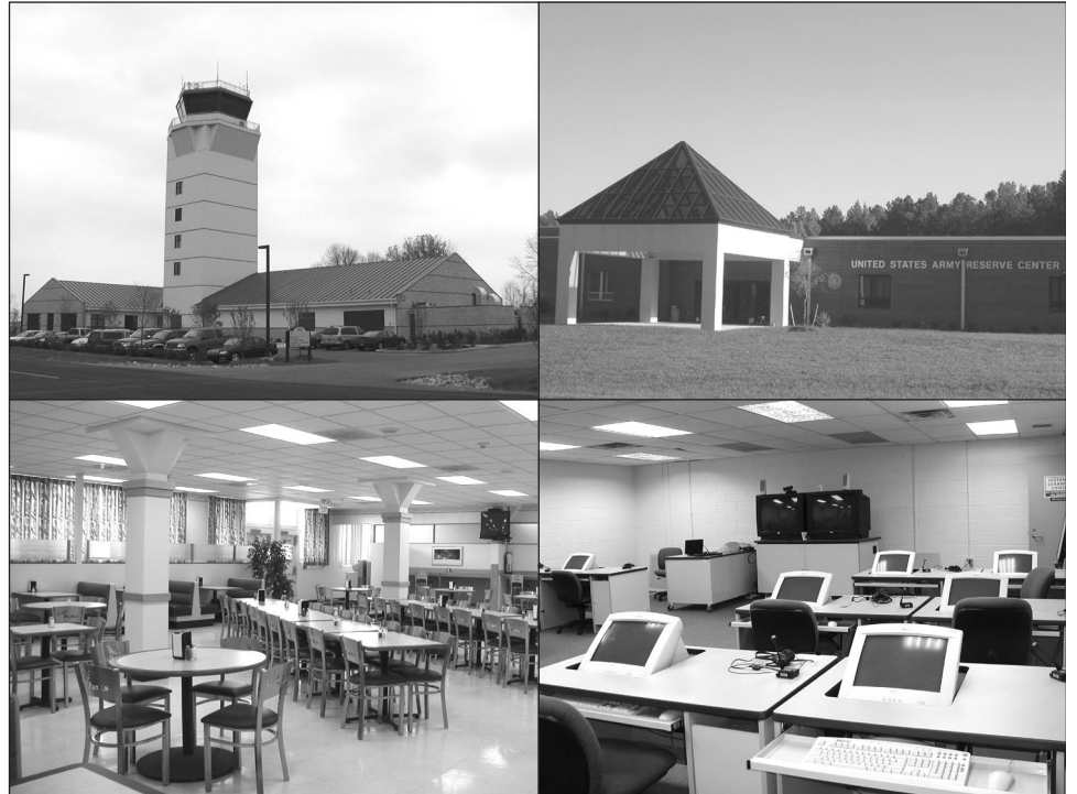
Figure 4: Typical Examples of Newly Constructed or Renovated Facilities at Various Reserve Component Locations
