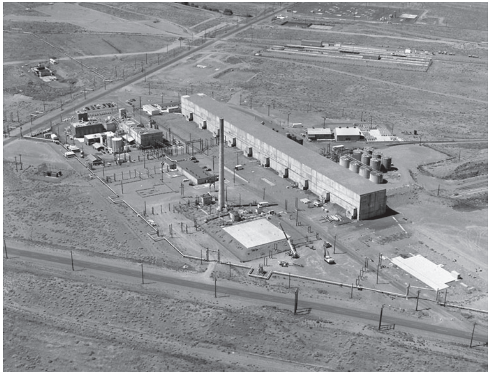
Figure 3: U-Plant at the Hanford Site, a Hazard Category 3 Facility
