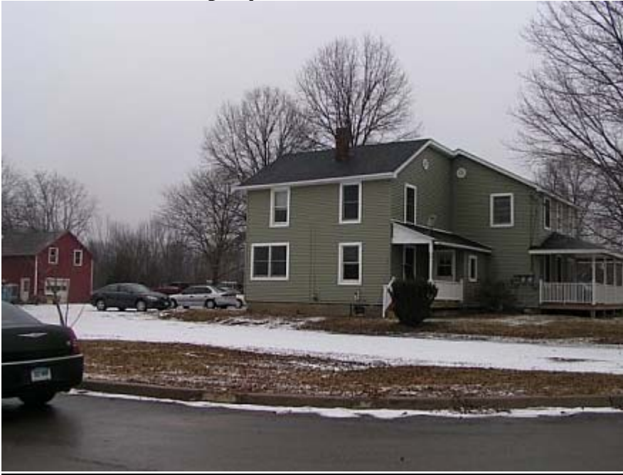
Vacant House on Property
