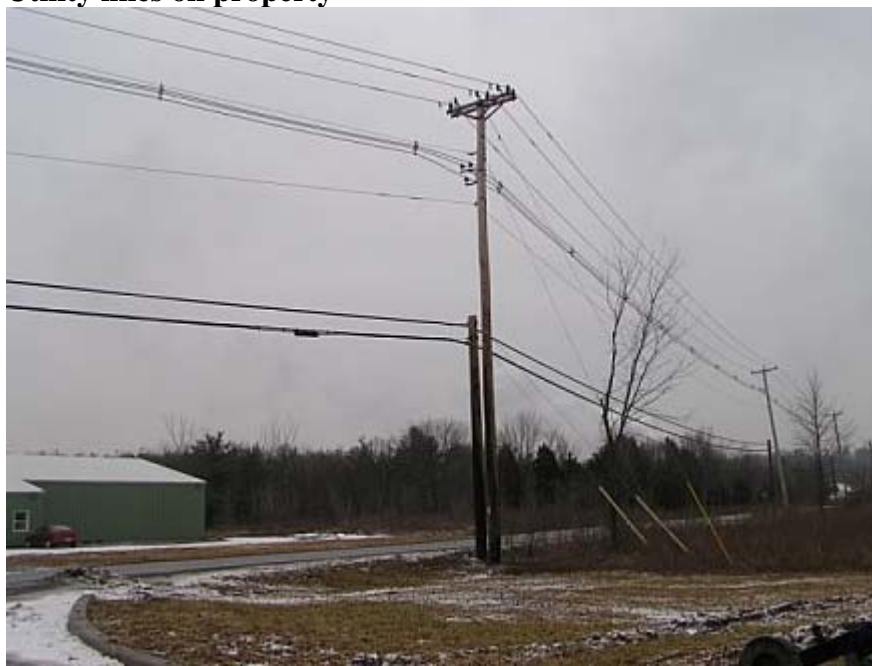
Utility lines on property
