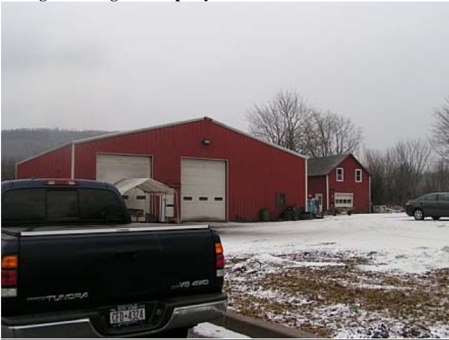
Storage Buildings on Property
