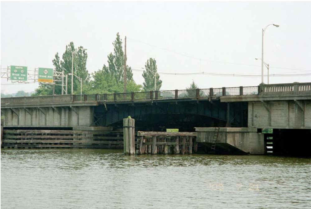
Route 46 bridge spanning Overpeck Creek
