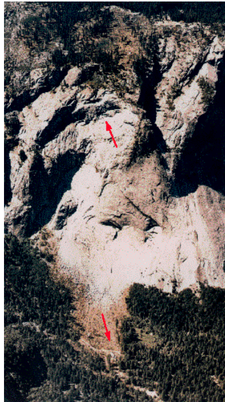
Figure 2. Rockfall below Glacier Point, Yosemite. Upper arrow shows source of rockfall; lower arrow points to the roof of the Happy Isles Nature Center, which is approximately 100 feet long.
