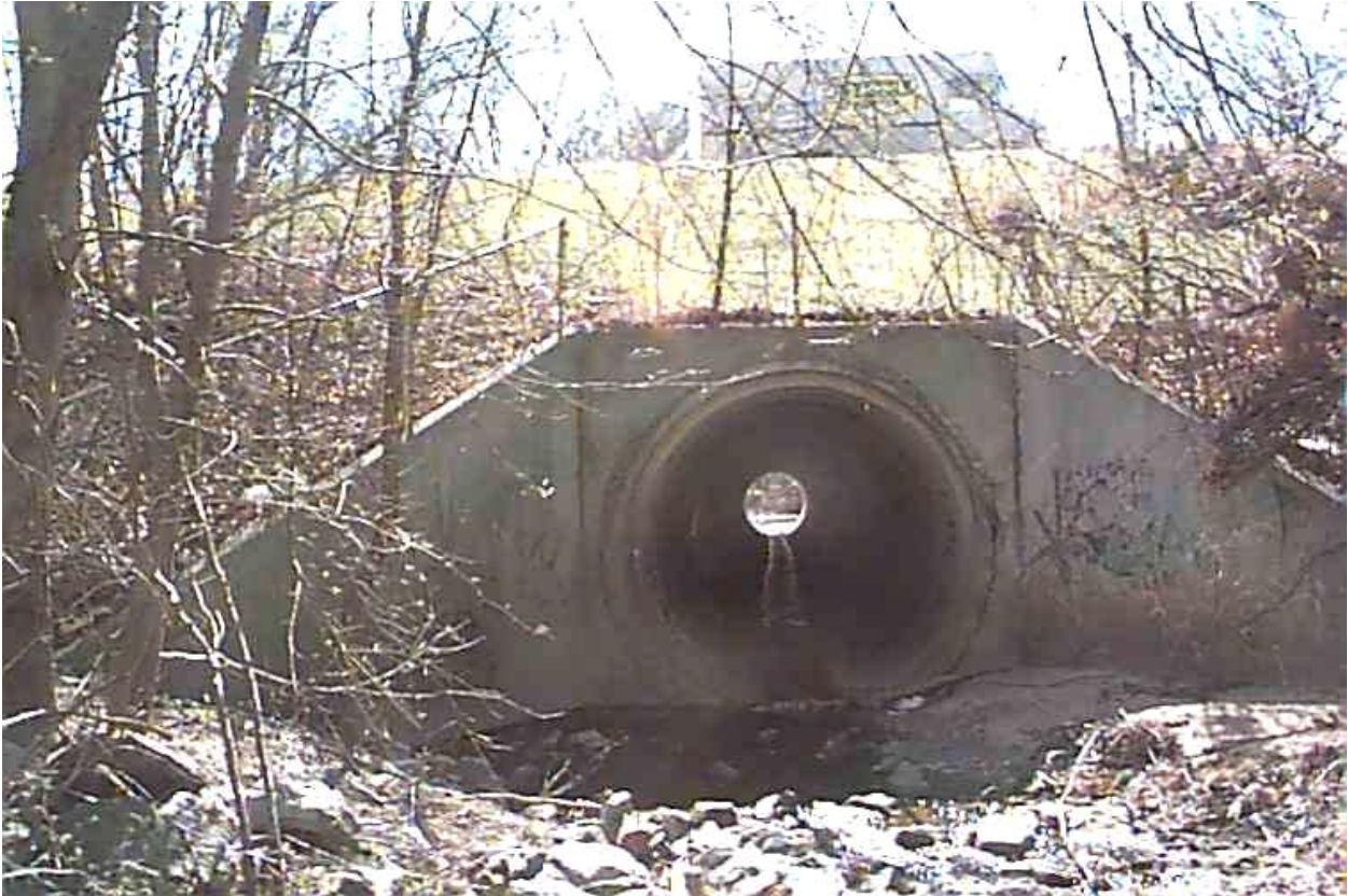
Figure 1. View of culvert looking downstream.
