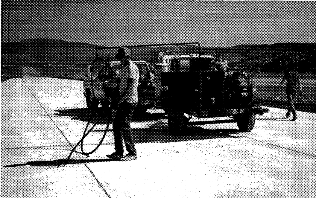
Figure 18. Hot-applied sealant installation at Heber City, Utah test site.
