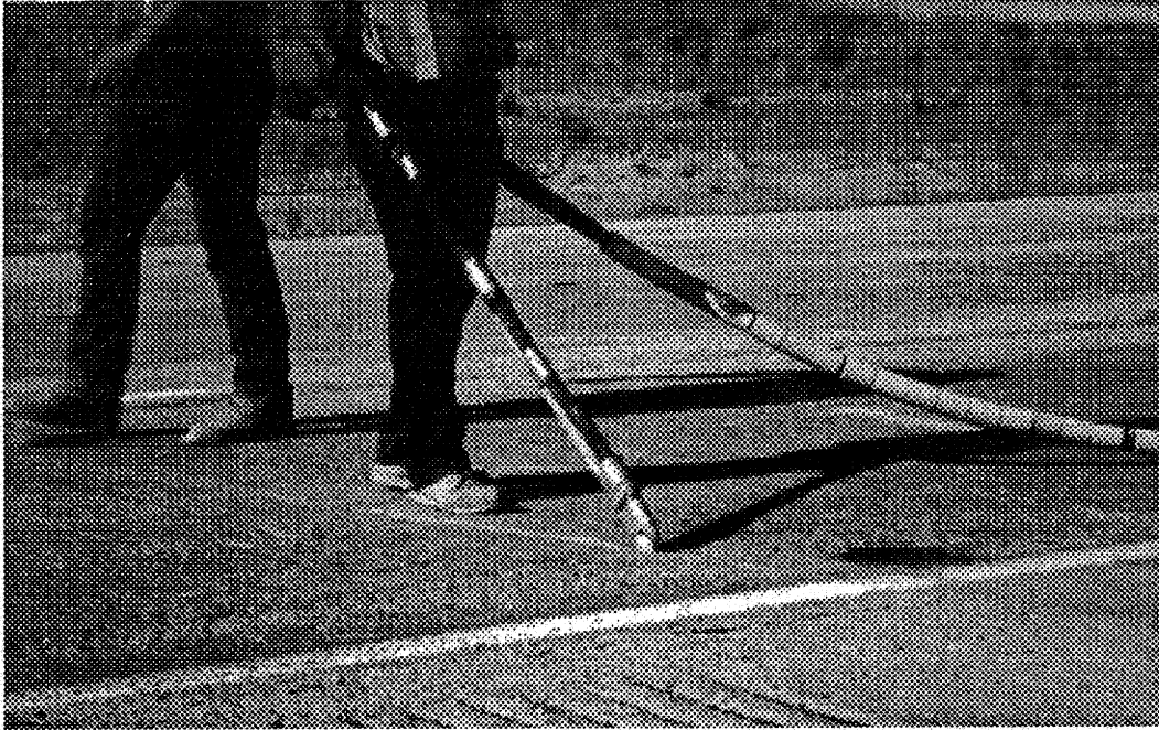
Figure 16. Sandblasting operation at Wells, Nevada test site.
