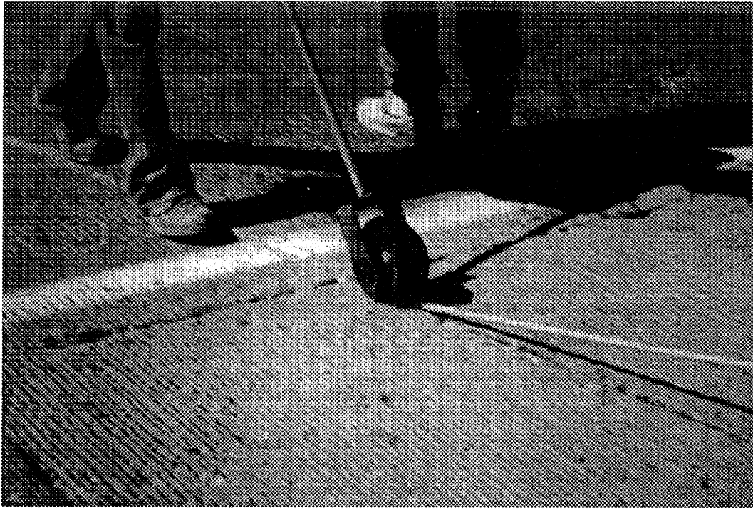
Figure 17. Backer rod placement at Campo, Colorado test site.
