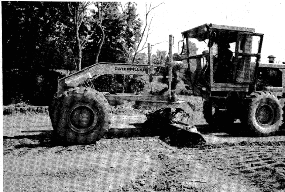
Figure 10. Grader-scarifier used in soil preparation.
