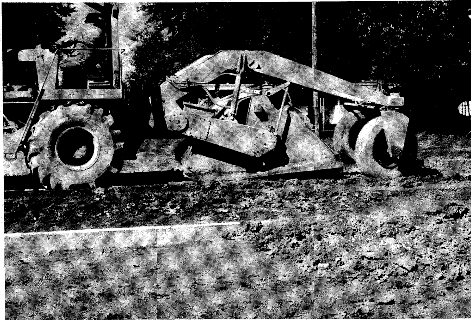
Figure 11. Rotary mixer used in soil preparation.
