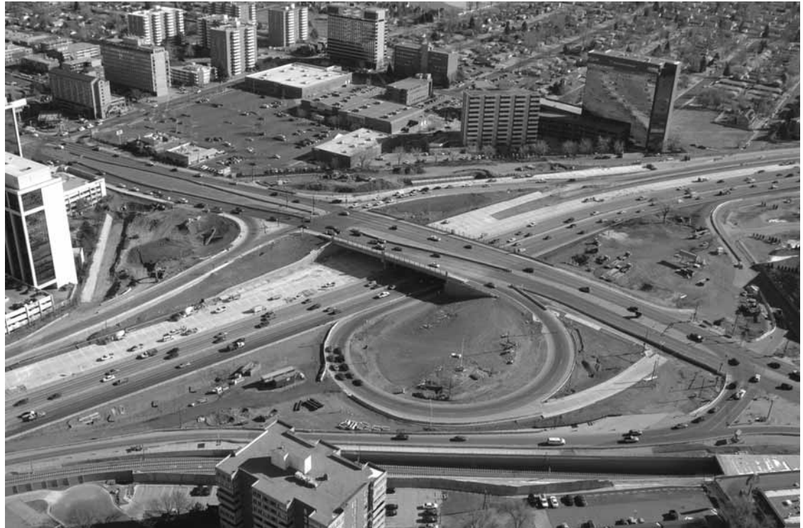
The T-REX project in Denver, CO, includes the reconstruction of 11 bridges spanning I-25. The Colorado Boulevard Bridge over I-25 was one of three bridges rebuilt in phases, so that traffic could be maintained on the structure at all times.
