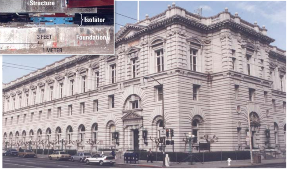
The 100-year-old Court of Appeals Building in San Francisco, California was retrofitted after the 1989 Loma Prieta earthquake using base-isolation technology (inset) and was fully reoccupied in 1996. Base-isolation systems dampen the shaking energy fed into the structure through its foundation, thus reducing the likelihood of damage. Sensors placed below and above the isolators allow measurement of the effectiveness of the system.
