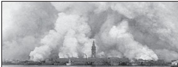
The fire that destroyed 500 city blocks after the 1906 quake raged out of control because liquefaction broke water pipes that were needed by firemen to fight the fire.
