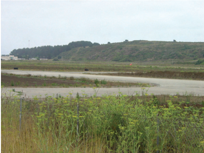
Figure 8-24. Scarp of the Seal Cove Fault, a strand of the San Gregorio Fault System, forms a linear ridge along the west side of the Half Moon Bay Airport.
