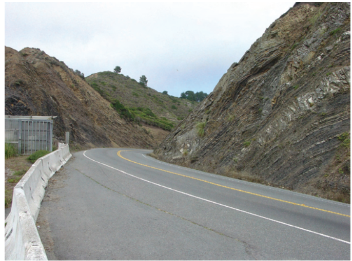
Figure 8-16. Road cuts along Highway 1 expose interbedded layers of Paleocene-age deep-sea-fan deposits (turbidites). This view is looking east from a small pull off at the top of the ridge of San Pedro Mountain. Note that this pull off is not recommended as a field-trip stop because of high traffic volume along the highway. Coastal travelers can more safely access similar deposits of Cretaceous age at Bean Hollow State Beach or near Pigeon Point south of Half Moon Bay.
