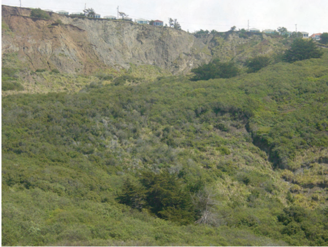
Figure 8-11. A massive landslide complex at Mussel Rock Park masks the main trace of the San Andreas Fault. Note the high, barren slump escarpment in the background. Ongoing coastal erosion at the toe of this slide area promotes the landward migration of the high wall of the landslide escarpment. Numerous homes have been destroyed, damaged, or condemned along this coastal slide area of Daly City.
