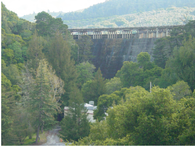
Figure 8-6. This view of Crystal Springs Reservoir Dam is from along Crystal Springs Road beneath the I-280 bridges over Crystal Springs Canyon. Skyline Boulevard crosses the dam. Sawyer Ridge is in the distance.
