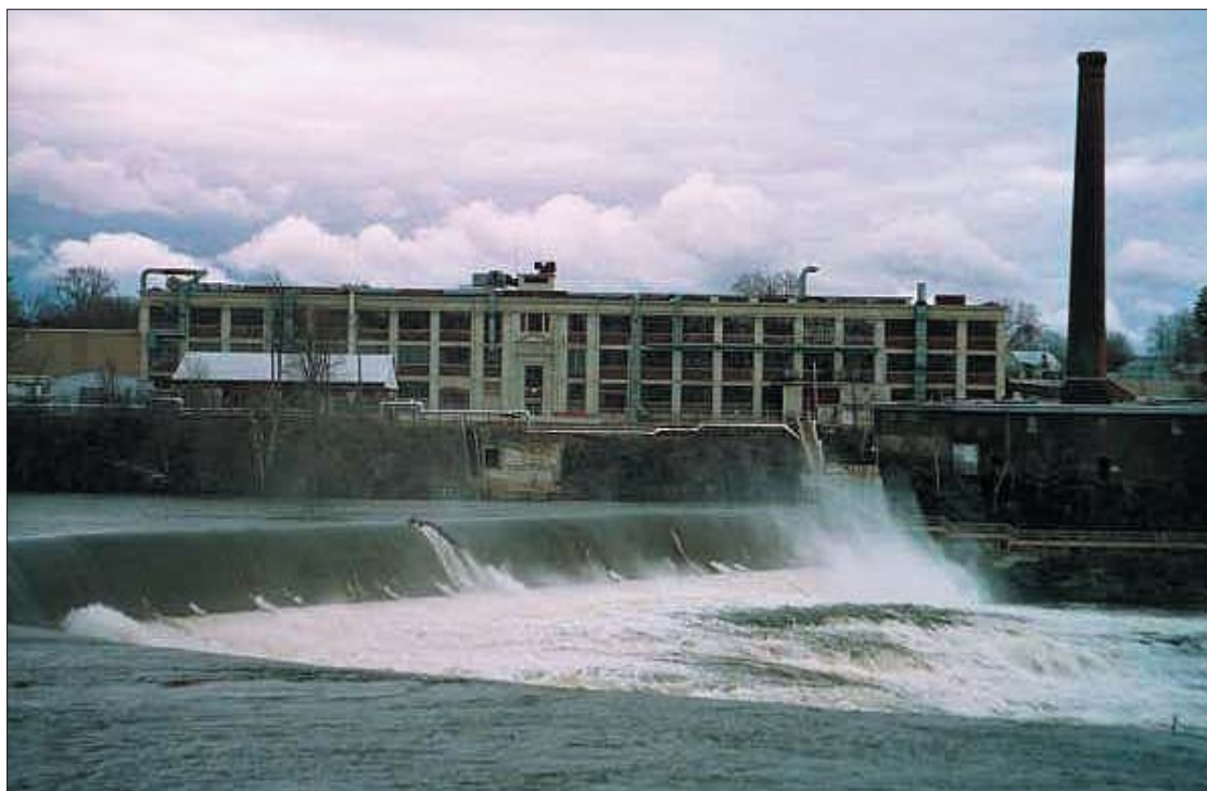
Hudson River PCBs site in New York where the group Scenic Hudson, Inc. used TAG funds to keep the community in Ft. Edward informed through newsletters and a Web site about the river cleanup. Source: EPA
