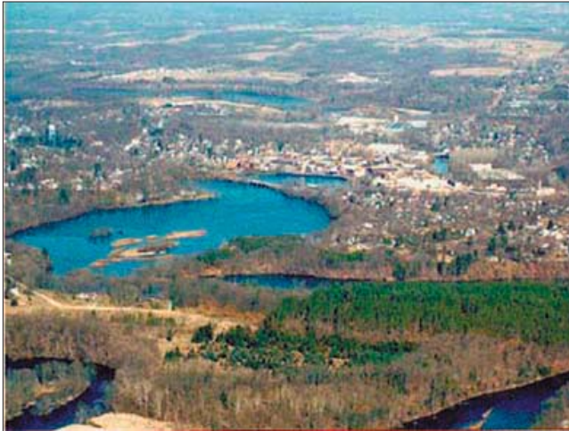
Aerial photograph of the Allied Paper, Inc./Portage Creek/Kalamazoo River area. Source: Michigan Department of Environmental Quality
