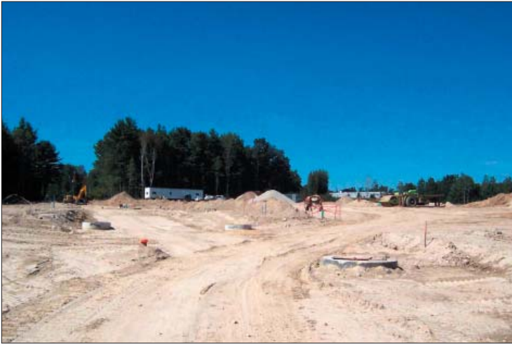
Construction at the Tinkham Garage site. Source: EPA
