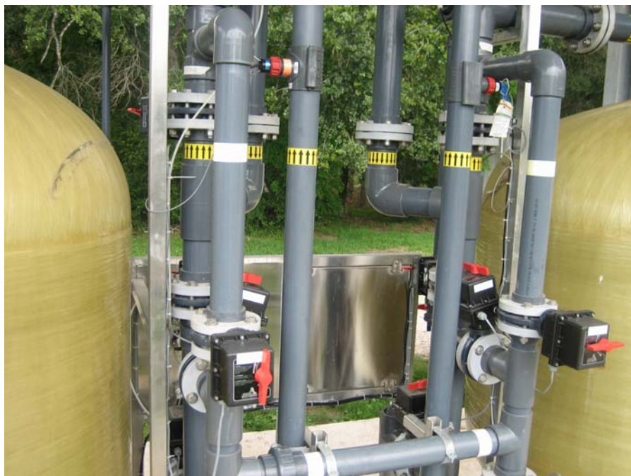
Figure 4-8. APU-30S System Valve Tree and Piping Configuration
