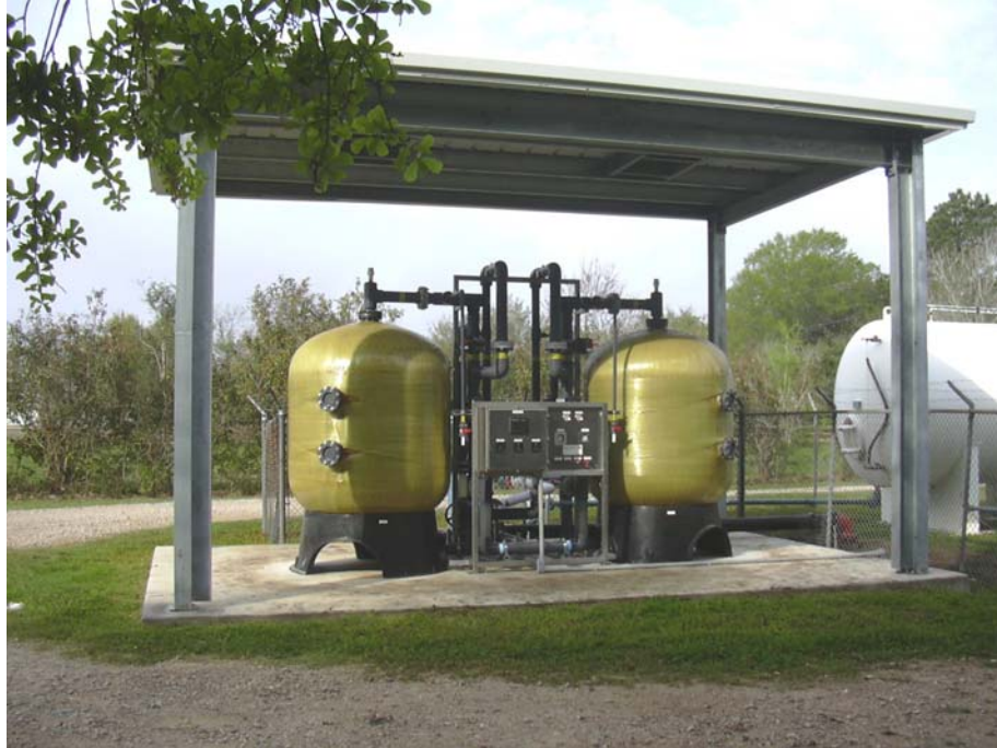
Figure 4-5. Photograph of APU-30S Arsenic Removal System
