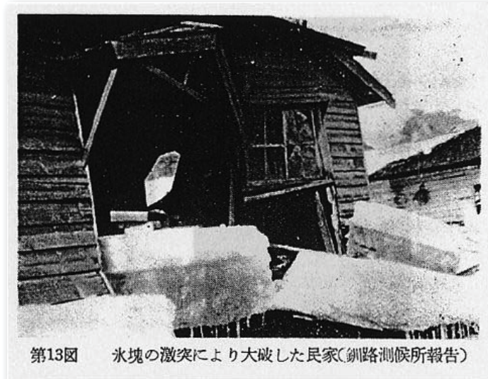
Large ice blocks entrained during runup of the 1952 Tokachi-Oki tsunami. Photograph courtesy of the Kushiro Branch of the Japan Meteorological Agency.
