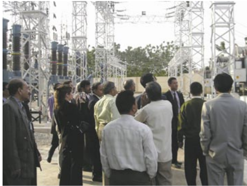
Andhra Pradesh Central Power Distribution Company representatives discusses operations and maintenance procedures with SARI/Energy executives from Bangladesh, Bhutan, India, Nepal, and Sri Lanka.
