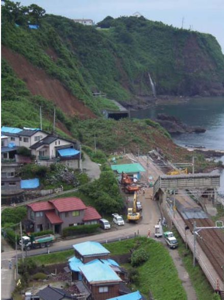
Landslide at the Umigawa train station.
