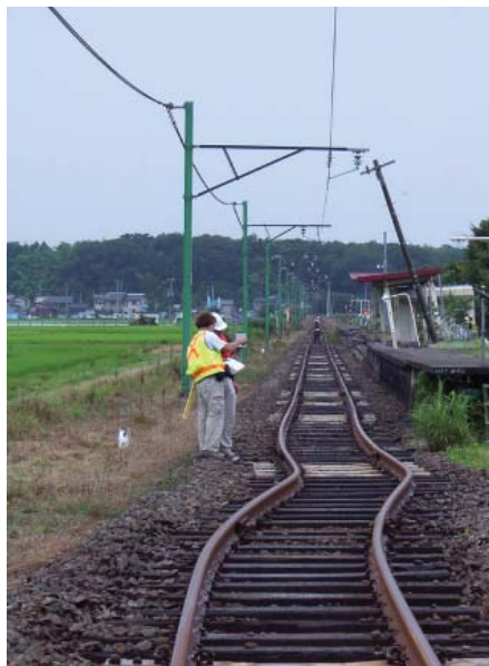
Permanent lateral deformation of train tracks at the Arahama station, the result of compression due to surface waves.
