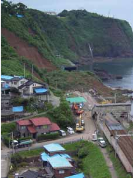
Landslide at the Uumigawa train station.
