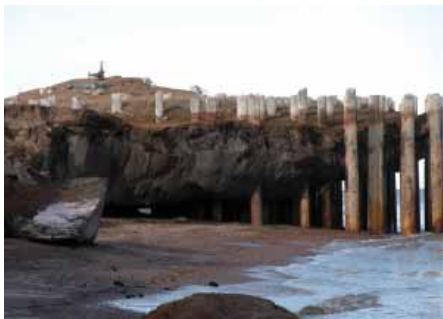
The rapid retreat of Arctic tundra coastline has exposed oil-exploration infrastructure on the shore of the Beaufort Sea, subject to some of the highest coastal-retreat rates in the world. Shown here are the wellhead and pilings of the J.W. Dalton Test Well #1 in September 2004 (left) and September 2005 (right). Drilled in 1979 as part of USGS exploration in the National Petroleum Reserve in Alaska, the well was originally located 1,500 ft inland from the Beaufort Sea coast; it is approximately 120 mi northwest of Prudhoe Bay. Photographs by Susan Flora , Bureau of Land Management.
