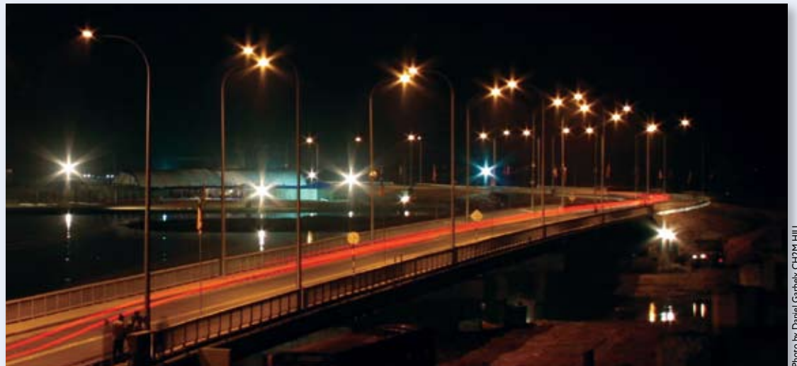
The new 185-meter long bridge across Arugam Bay links three ethnically diverse communities on the coast of eastern Sri Lanka, in a region well known for its beautiful beaches.
