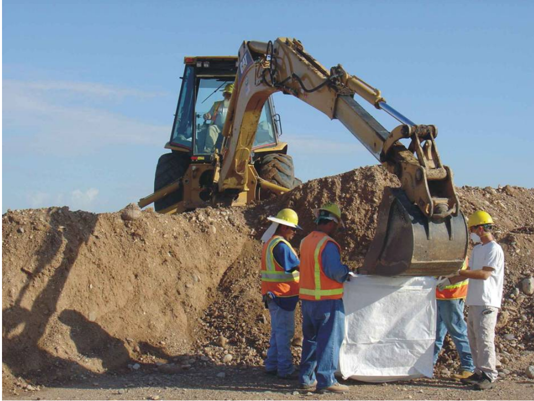
Figure 2-1. Collection of Arizona Soil Bulk Sample
