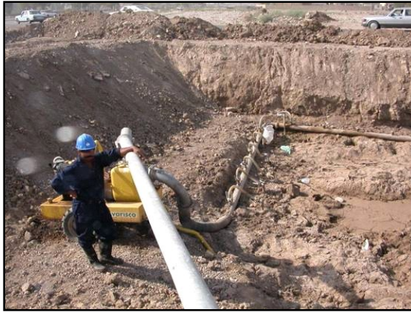
Draining work to rehabilitate a Baghdad sewage system
