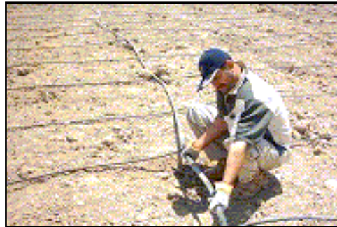
Drip irrigation system installation
