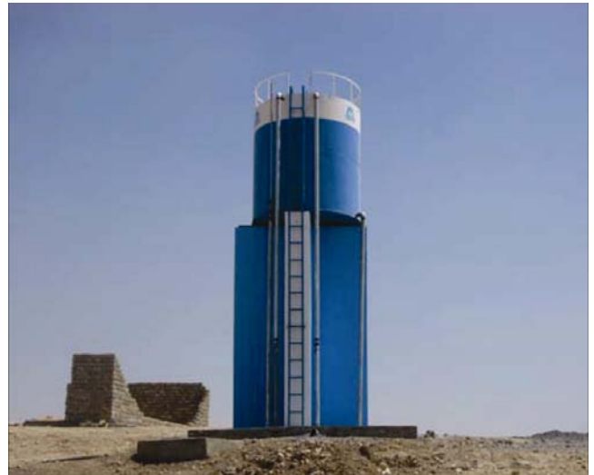
An elevated water storage tank constructed in the Arbil Governorate is part of a larger system providing safe, potable water to a series of villages in the region.
