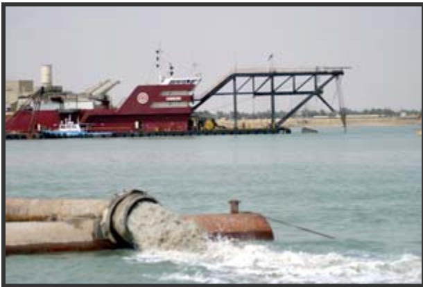
Output pipe from the Carolina dredging vessel, at the port of Umm Qasr. (photo: Bechtel)
