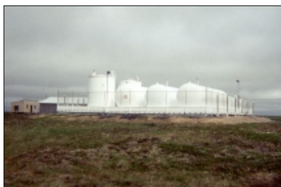
Tank farm after upgrades.
