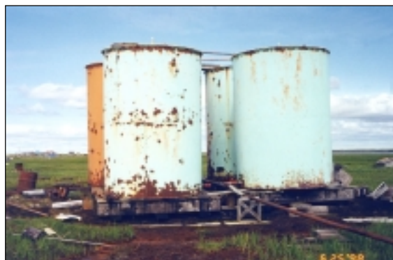
Tank farm before upgrades.
