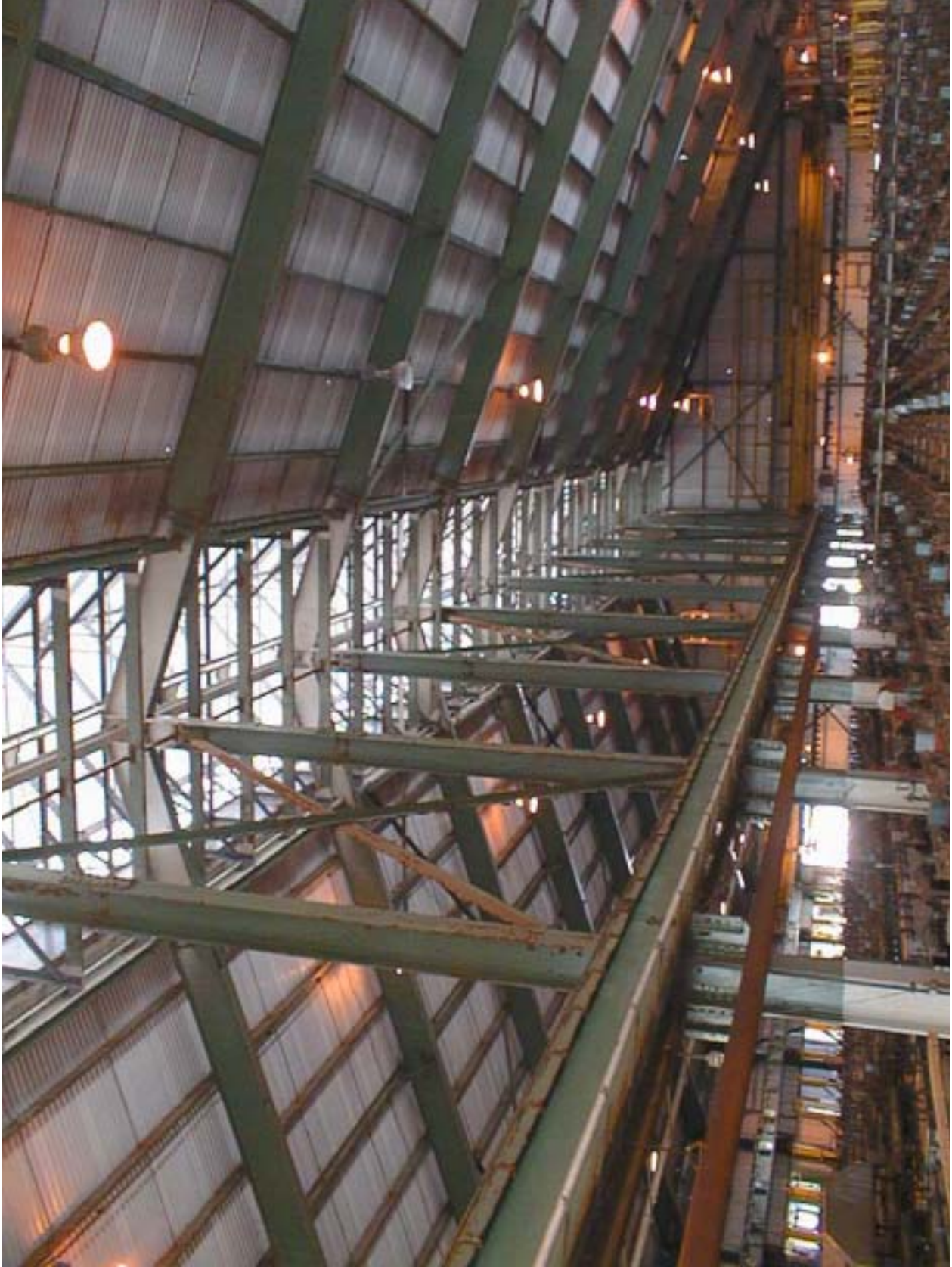
Figure 3-3a. Cell building showing interior of roof ventilator.
