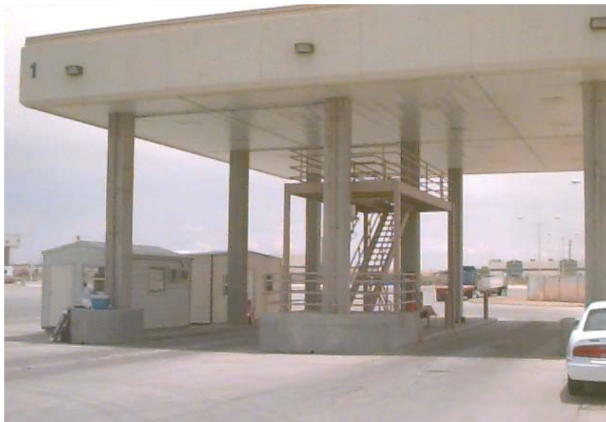
Figure 9. Inbound safety inspection checkpoint beside primary on the U.S. side.
