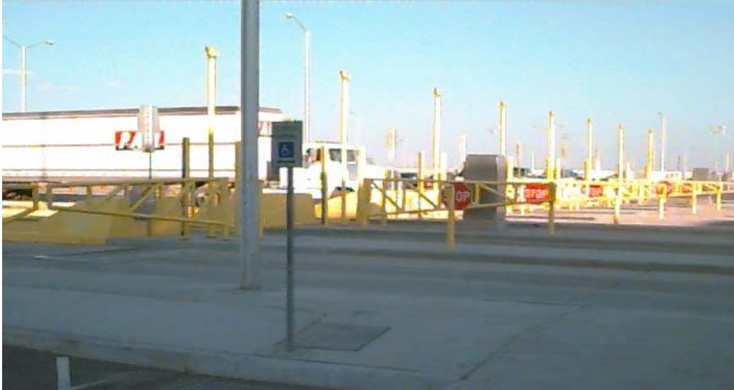
Figure 5. Outbound Toll Booths at the World Trade Bridge
