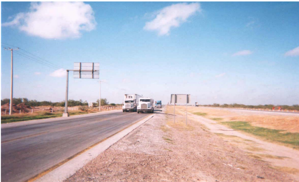
Figure 8. Access Road Approaching the World Trade Bridge in Nuevo Laredo
