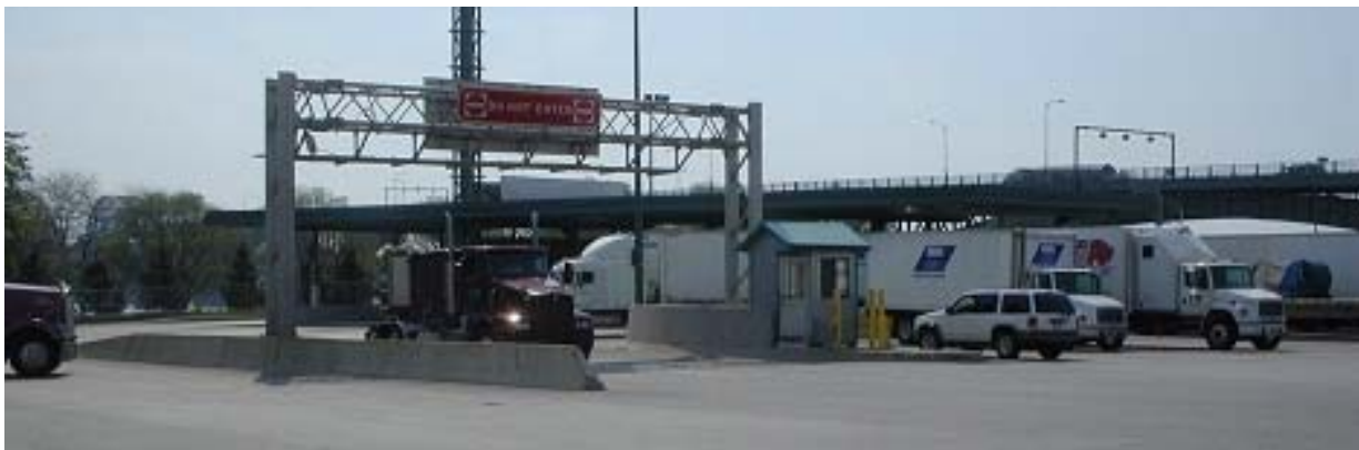
Figure 5. Canadian Customs Primary Inspection Booths, Showing the OB-2 Collection Location
