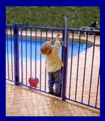
Install a self-closing, self-latching gate that opens out, away from the water.
