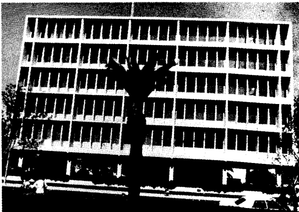
FIGURE 9.—Imperial County Services Building, El Centro, Calif., which suffered significant structural damage during the 1979 Imperial Valley earthquake. View north.
