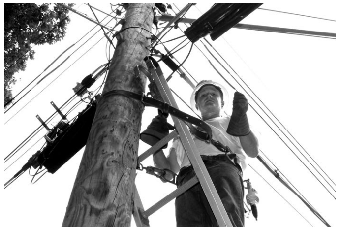
Line installers and repairers wear safety gear to protect themselves from electrical current.
