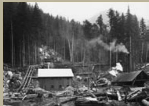
Skagit Dam construction site, 1921
