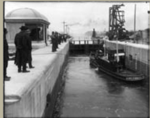
Ballard locks under construction, 1916
