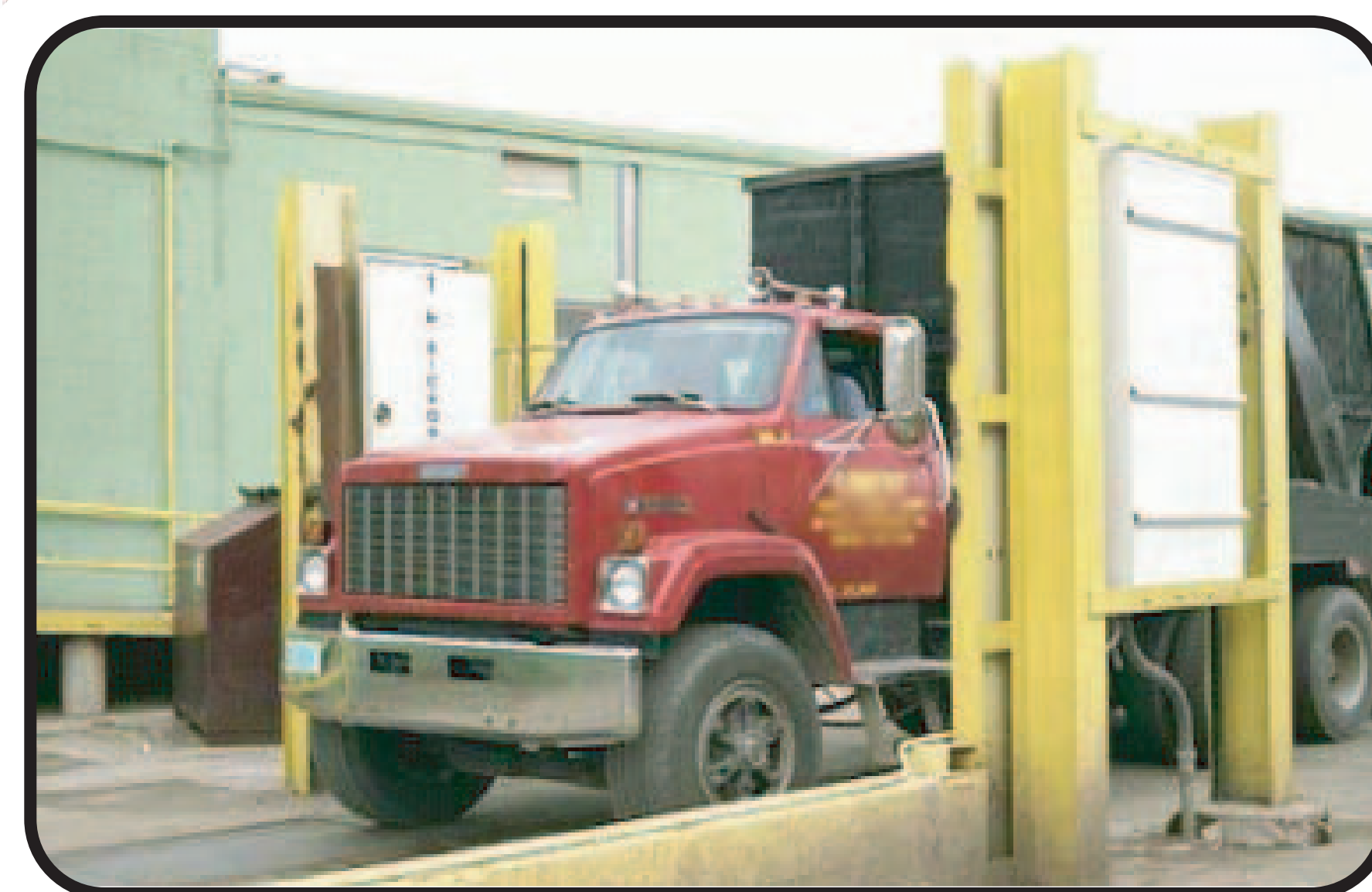
Portal Radiation Monitors at Scrap Yard
