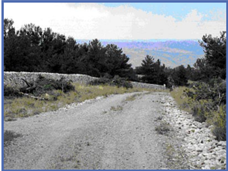
Access road being treated.
