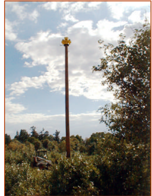
The warning siren installed to alert residents to evacuate if necessary.
