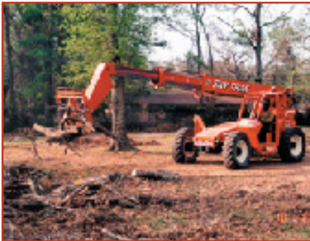
Jackson Hotshots helping to remove debris from a Panama City neighborhood hit by hurricane Frances.
