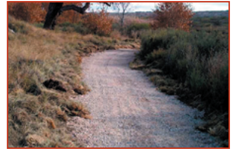
Existing trail widened to serve as a fuel break for the prescribed burn at the draw.
