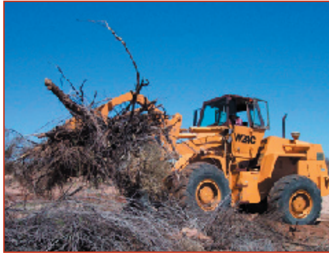
A grapple rake attached to a loader was the extraction method used at the Overflow Wetlands Area of Critical Environmental Concern.
