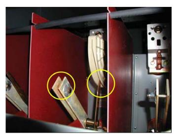
Improperly maintained switch may result in arc interrupter blade not fully open from arc chute and may still conduct current with the handle in the open position.
