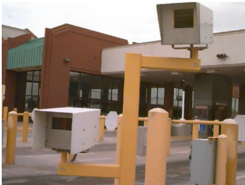
Figure 7. License Plate Reader at the Zaragoza Bridge, El Paso (Automobile Side)
