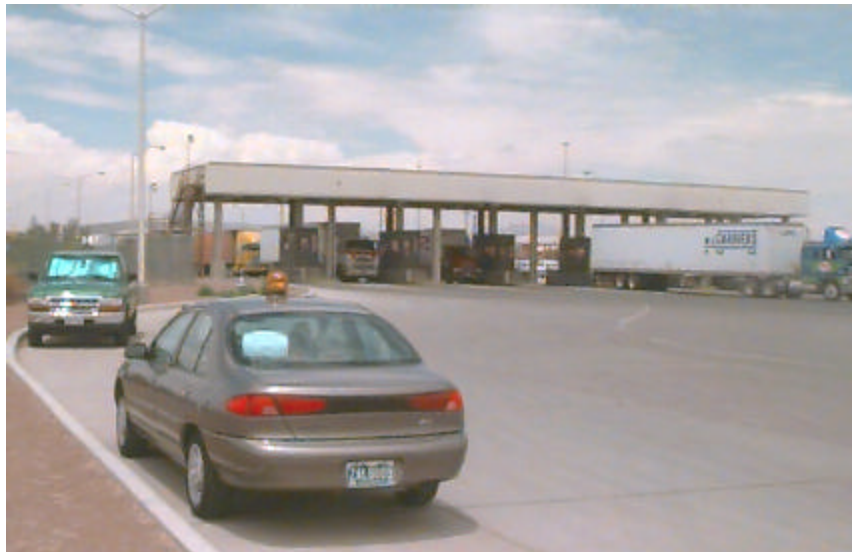
Figure 4. Primary on the U.S. Side of the Zaragoza Bridge (El Paso-Juarez)
