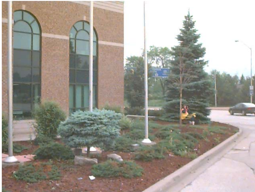
Figure 15. Outbound 2 data collector beside Canadian Customs building.
