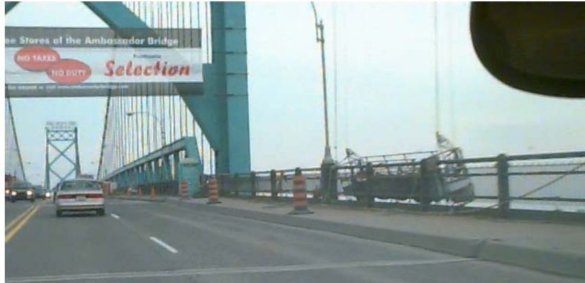
Figure 2. Maintenance Equipment on Ambassador Bridge.
