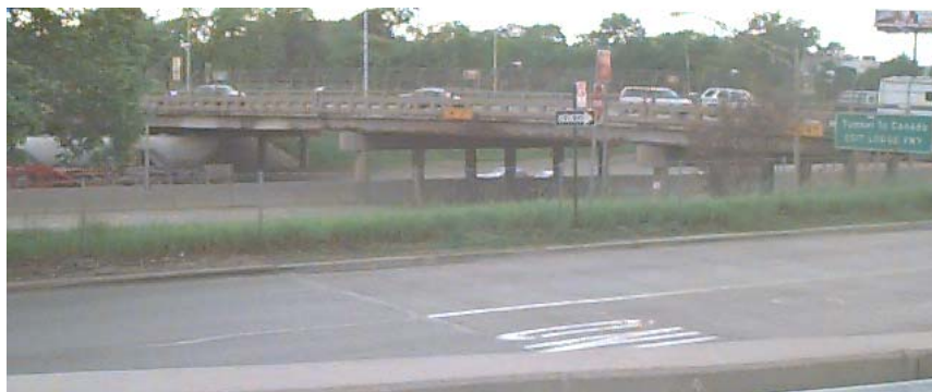
Figure 12. Outbound traffic crossing the Porter Street overpass above I-75.
