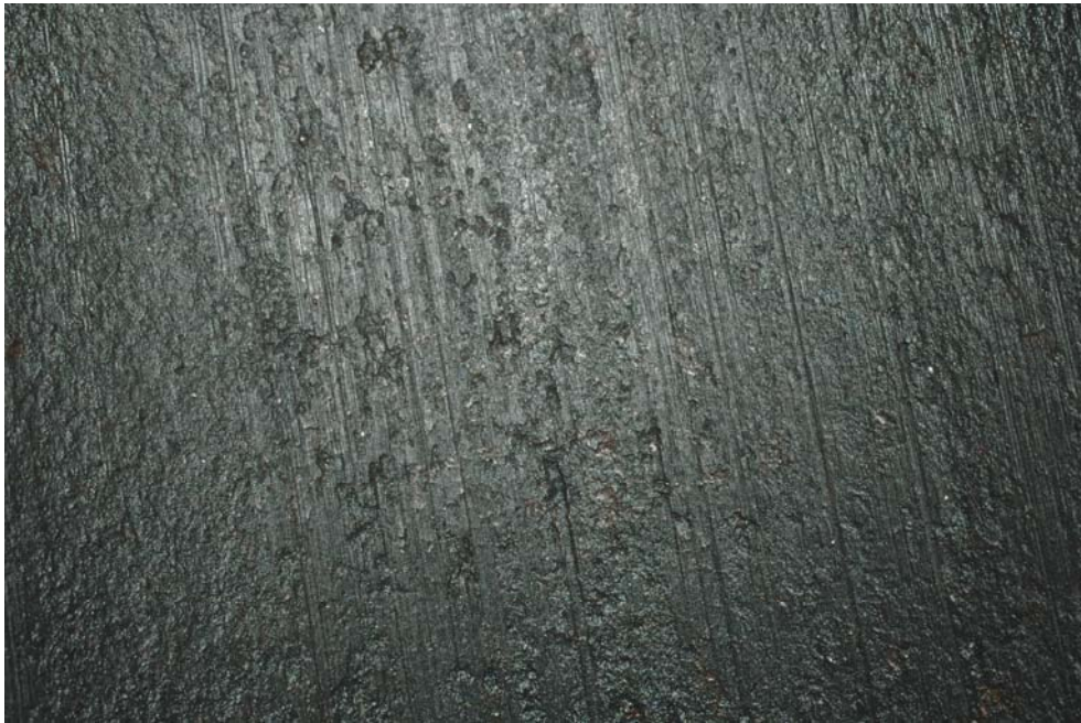
Figure 3: Inside surface of the DOT-3AA cylinder. No major corrosion observed.
