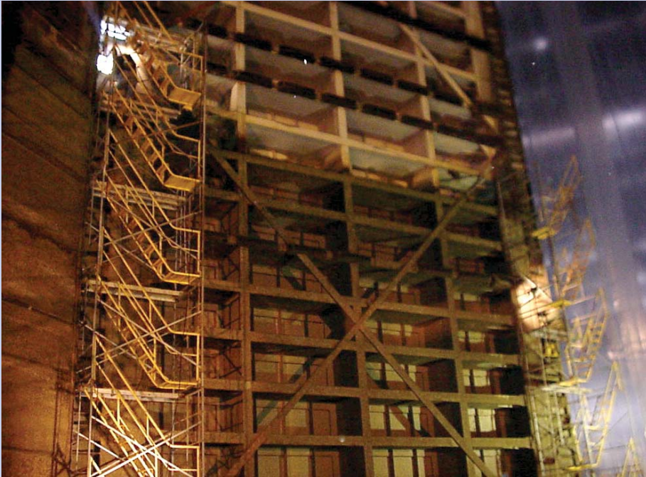
MVC-788 Downstream south miter gate leaf setup for crack welding.
