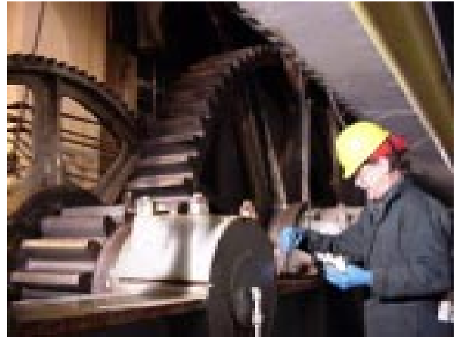
Trades Helper Larry Cheney inspecting and lubricating culvert valve open gears.
