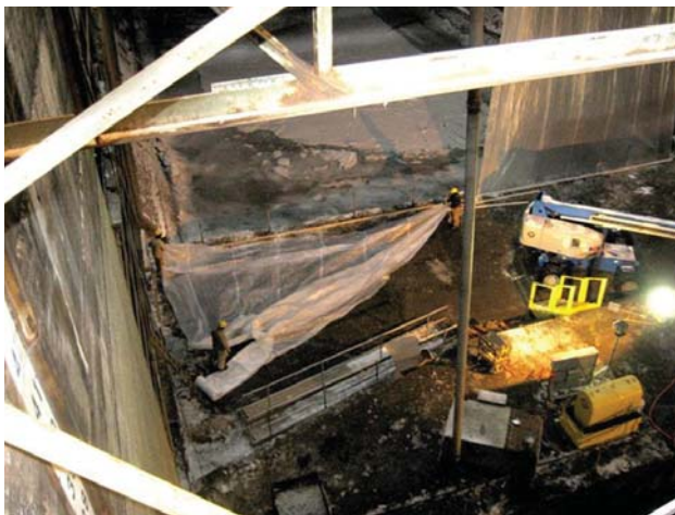
Crews hang plastic curtains to isolate the work area.
