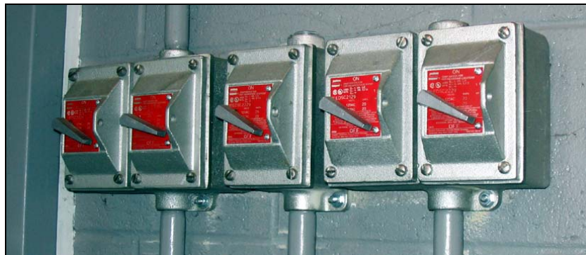
Figure 28. Explosion Proof Switches
