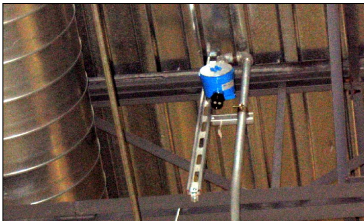
Figure 27. Hydrogen Detector Located at Ceiling Level
