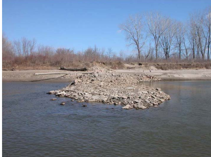
Figure 19. Example of unrooted dike that has been knocked down and flattened to create habitat. These low-angle engineered deposits may mimic naturally occurring particulate spawning substrate.
