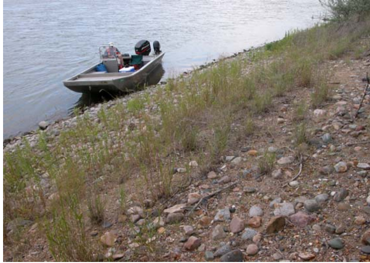
Figure 7. In-place glacial drift located on the right descending bank downstream from the Highway 81 bridge, near Yankton, South Dakota
