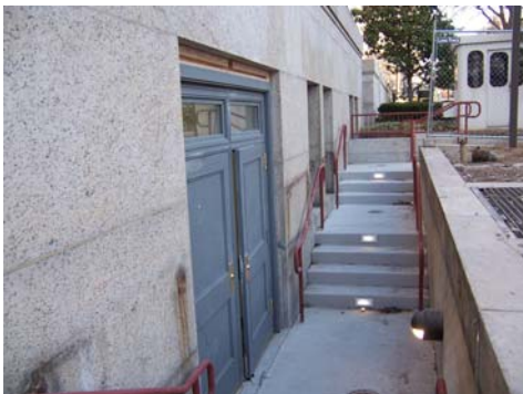
18th Street Exit discharge
